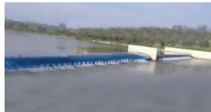
Rubber dam in Hetian, Xinjiang
