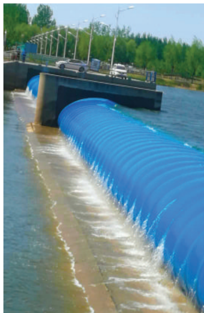
Liaoning Pu ruver rubber dam
