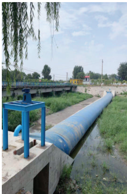
Fengfeng coal mine rubber dam
